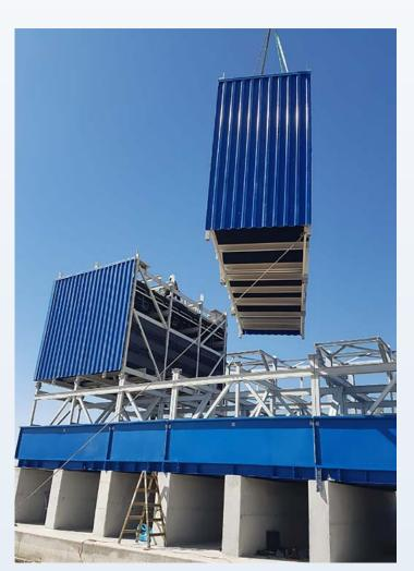
YWCT developed a medium size cooling tower (600 m $^3$ /hr – 2,000 m $^3$ /hr per cooling tower) made of pultruded FRP with integral FRP basin. The cooling tower is delivered to site in modules which reduces installation time on site to few days instead of weeks.
